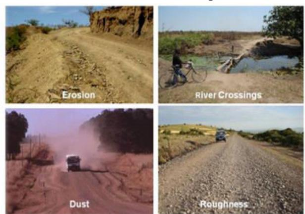
Figure: Typical problems are gravel road networks
