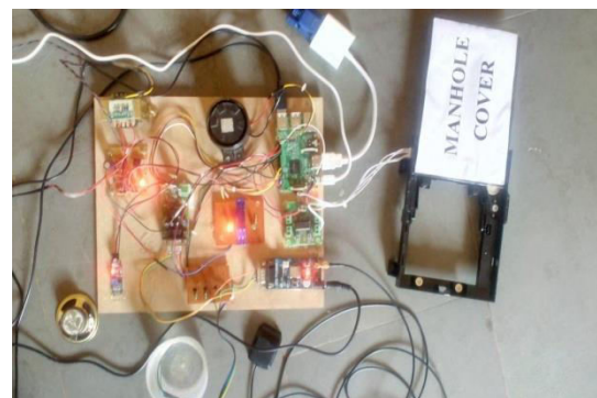
Figure 5.2: Opening Manhole Cover when the water level crossed the cut-off value.
