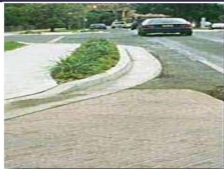
Figure 1.2: Application of Recycled Aggregate as Road Kerb (Source: Building Innovation & Construction Technology, 1999)
