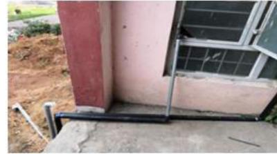
Figure 3.5 Insulation for Galvanized steel pipes
