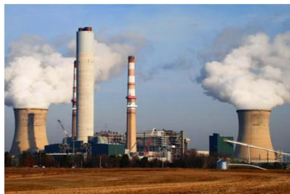
Fig: 1 Fig. 1 shows a photograph of self-supporting steel chimneys located in an industrial plant.
