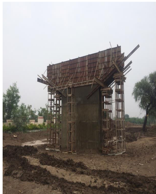
Shuttering work at project site
