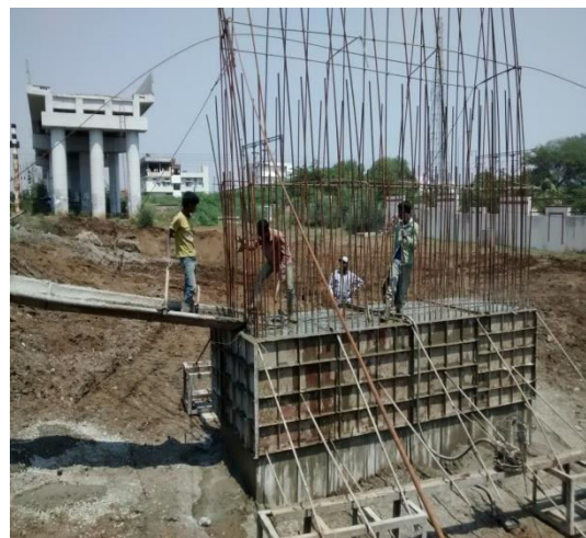
Casting work at project site
