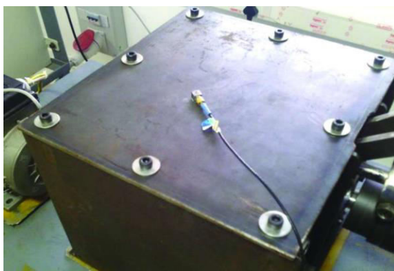
Fig 3.2 Accelerometer placed on gearbox casing
