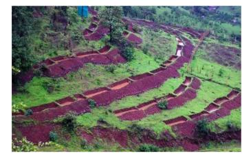
Deep Continuous Contour Trenches are an advanced version of CCTs designed to capture and store a larger volume of rainwater. They are deeper and wider than regular CCTs, allowing for increased water storage and infiltration. Deep CCTs are especially useful in areas with high rainfall variability and are effective in increasing soil moisture levels, benefiting agriculture and vegetation.
