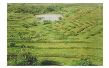
Continuous Contour Trenches are water harvesting structures commonly used in hilly or sloping terrains to conserve rainwater and reduce soil erosion. They are typically trenches dug along the contour lines of the
