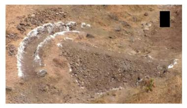
Small earthen dams are constructed across seasonal or intermittent streams to impound water during the rainy season. These dams are typically made of compacted earth and are designed to store water for various purposes, including irrigation, livestock, and domestic use. Small earthen dams are a simple and cost-effective way to capture and store rainwater, providing a valuable source of water in arid or semi-arid regions.
