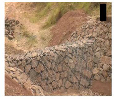
Gabion structures are made of wire mesh baskets filled with stones or rocks. They are commonly used in water harvesting projects to control erosion, stabilize slopes, and create check dams. Gabions slow down the flow of water, allowing sediment to settle and water to infiltrate into the ground. They are versatile and can be used in various terrain types, making them a valuable tool for water conservation and land management.
