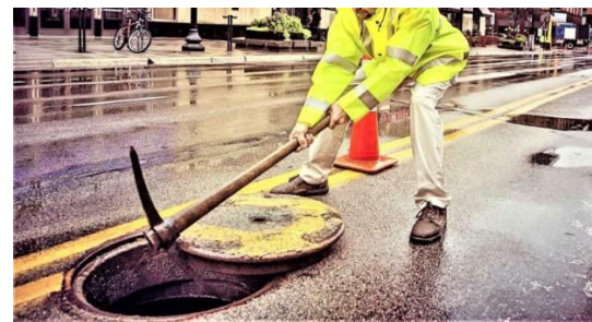
Figure 1. Manual checking of manholes
