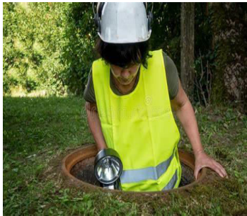
Figure 4. Manual Monitoring of manholes
