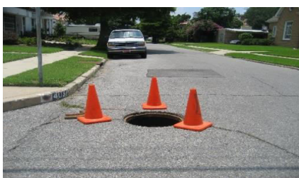
Figure 5. Traffic zones around open manholes
